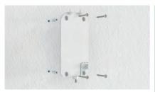
Fix the bracket to the wall using the screws supplied, taking care not to deform it.
