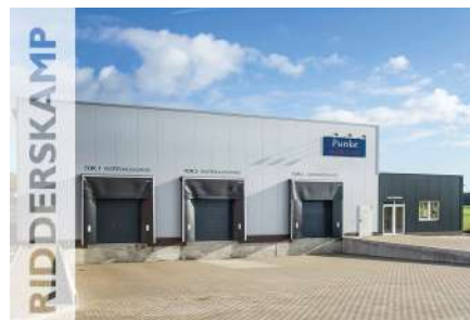
Warehouse and Service Centre
