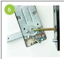
Use the spindle of the inside unit to turn the mechanism clockwise for as far as it goes. Make sure the spindle is all the way in.
