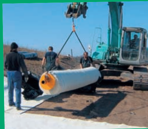
Fig. 2 Bentofix® capping installation
