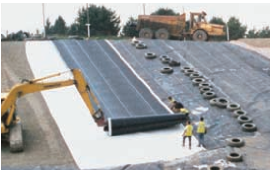
Geomembrane installation over GCL
