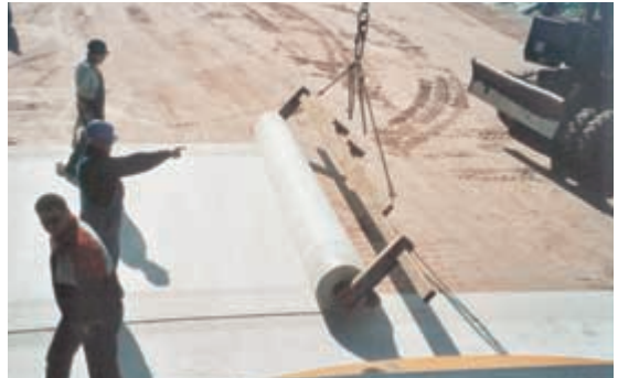
Bentofix® installation
