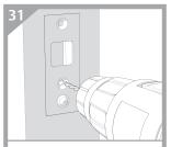
Drill Ø2mm pilot holes, affix with screws provided.
