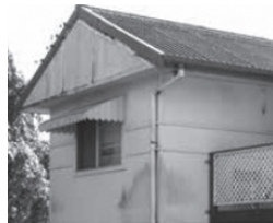
Asbestos Wall Sheeting
