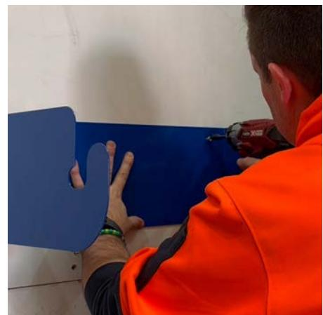
1. Place dispenser frame at desired height (ensure level) and mark holes for drilling.
