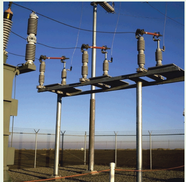
FIGURE 1. Transformer protection using SMD Power Fuses.
