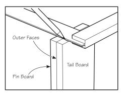
Figure 21: Marking the dovetail locations with a square. Extend the lines completely across the ends.
