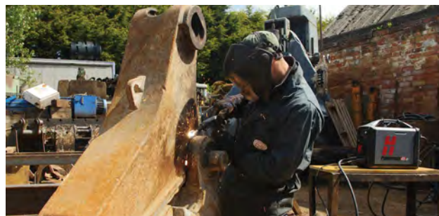
Maintenance and repair
